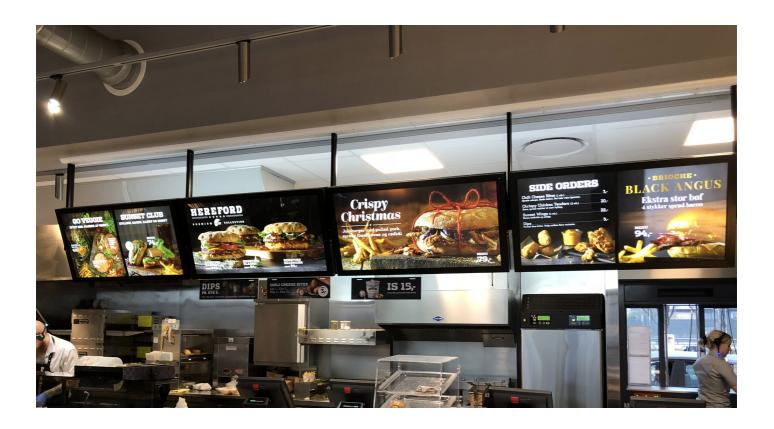
An appreciated menu system that has been used as standard by several fast food chains and gas stations. The double-sided reversible menu board have a fixed 40 mm wide profile at the top and on the sides and an openable profile at the bottom. The light box image and the protective plastic are pressed in under the openable profile when changing the image. Then the profile is closed.
